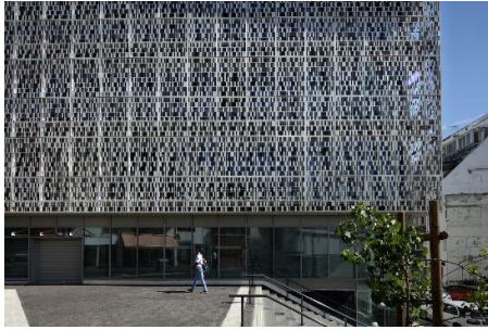
[4] C1 office block at Grand Chemin, Saint-Denis – example of effective double-skin architecture
