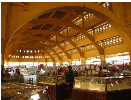
[3] Phnom Penh covered market, an example of tropical shelter architecture.
